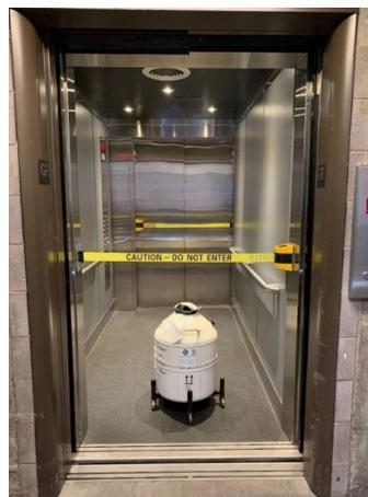
Figure 1. The elevator is taped off for transferring liquid nitrogen
